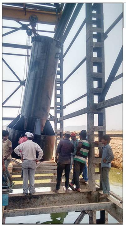
Uniquely designed Free standing Bottom Canister stand rested on the sump bottom without any fasteners to avoid imposing thrusts on the fragile MS floor of existing pump room.
