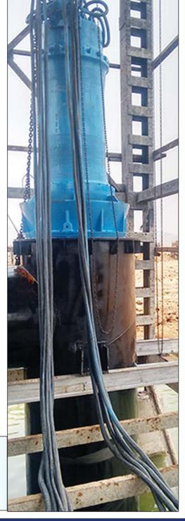
ATB pump has been lowered to the Canister-Tube, which would be rested on the canister ring which is in turn rested simply by bottom resting on sump without any foundation/ holding bolts/ fasteners.
